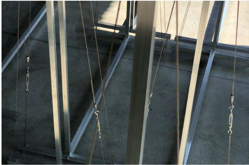
8.8 The wires are tensioned using a turnbuckle.
