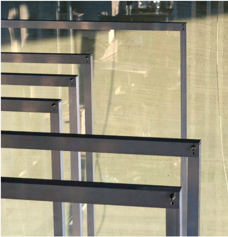
8.6 Top detail of the wire connection.
